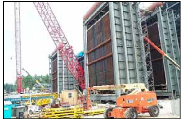
AES Granite Ridge Plant under construction in Londonderry, NH
